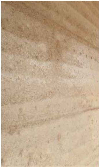
rammed earth wall (earth color)
