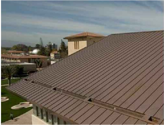
metal roof sheeting (copper)
